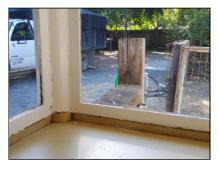
We observed "untempered" (not laminated safety glass) glass in some of the windows that are less than 18 inches above the floor, and in some of the older door glass. This is typical in homes of this age, however it could be hazardous if broken. Upgrading these locations should be considered for maximum safety.
