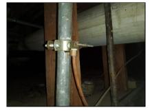
The galvanized steel water supply lines were corroded and the water was rusty or discolored at some of the fixtures. This is usually from mineral deposits building up inside of the older galvanized lines, particularly if fixtures
