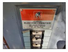
One of the screws was missing from the main electrical panel cover. We recommend replacement with an approved blunt-end screw to prevent movement and for improved safety.
