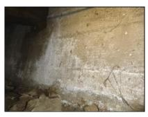
We observed exposed rebar visible within the concrete foundation at the left side, under the left side hall bathroom, as seen from the crawl space, where it appears the stemwall had been cut to accommodate the tub drain. We recommend that the exposed rebar be wire brushed, primered and sealed to prevent corrosion, expansion and subsequent damage to the concrete foundation.
