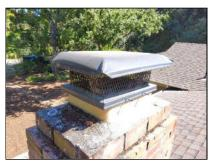
The mortar cap at the top of the chimney (also known as the crown wash) was cracked, eroded and/or poorly sealed. This is a common condition, but can lead to moisture penetration and subsequent damage. We recommend that it be resealed by a chimney specialist as a preventative measure.
