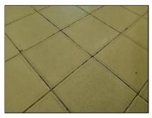
The flooring at the base of the right side hall shower was poorly sealed. We recommend that the floor be recaulked to help prevent moisture penetration and subsequent damage.
