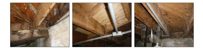
A there was no subfloor insulation installed in the subarea. Upgrading should be considered for improved efficiency.
