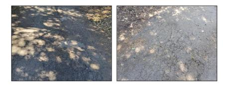
There was cracking and settlement observed in sections of the brick walkways at the right side. We recommend patching or repair for improved appearance and safety.
