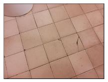
There were gaps or voids noted in the grout between some of the floor tiles in the left side hall bathroom. We recommend regrouting and/or caulking to help prevent moisture penetration and subsequent damage.
