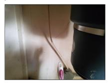
★ We observed an uncovered electrical junction box in the utility basement, above the water heater. We recommend that it be fitted with an approved cover plate to protect the wiring from accidental contact and physical damage.
