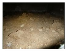
Left over construction debris has been left under the building. We recommend all debris be removed for improved access and reduced pest-related activity.
